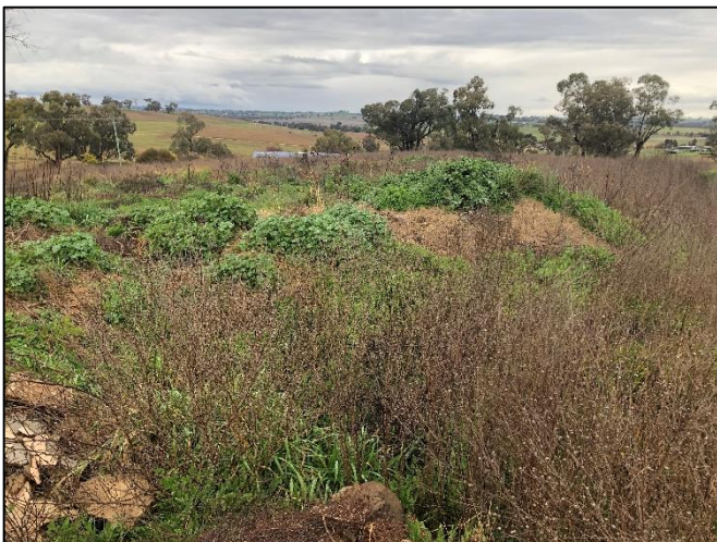
Stockpile 1 from site cleanup
